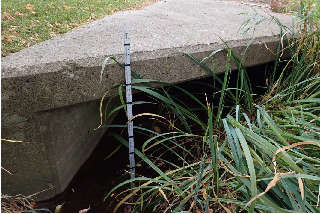
Highway 6 Concrete box culvert at the upstream extent of TBC-1
