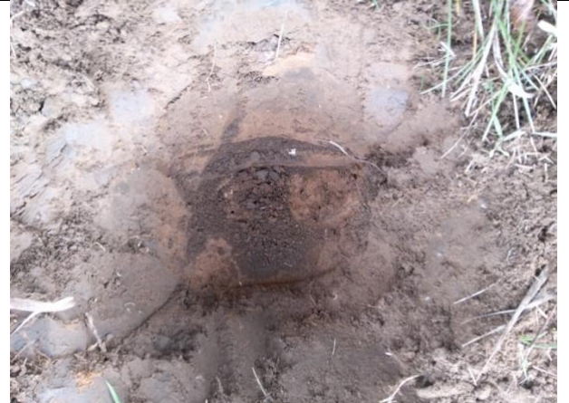
IMAGE 6 VIEW OF COMPLETED TEST PIT
